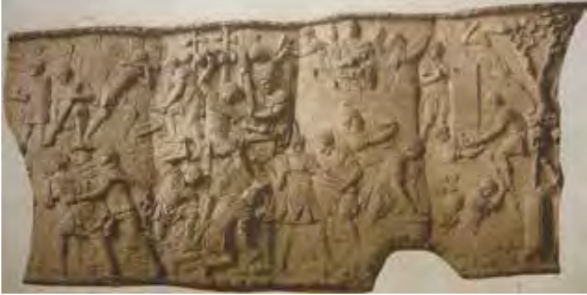
Trajan's Column (Cichorius Plate) Scene 19 (center): Building a Bridge
